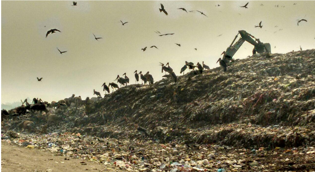
Open uncontrolled pathetic condition of the dumpsite
